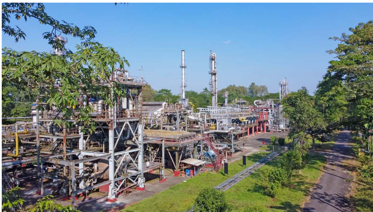
BCPL Lakwa Plant
